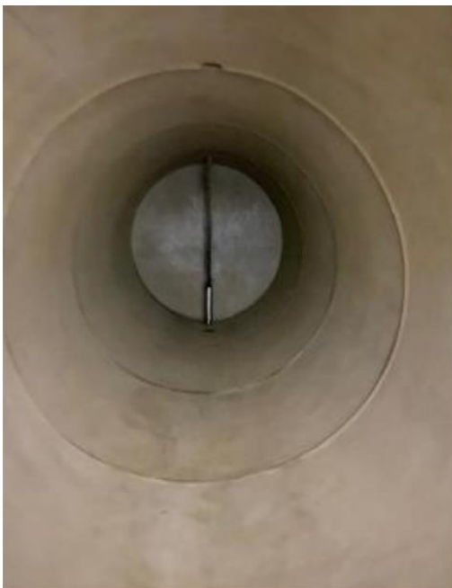
Before Lining, After Sandblasting
