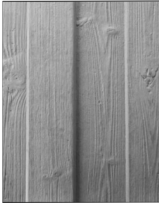
POUR-IN-PLACE RETAINING WALL (MATCH ARCHITECTURE GARAGE WALL FINISH)
