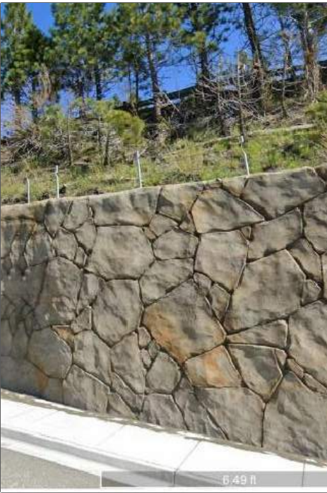
SOIL NAIL WALL (STONE-FACED CONCRETE FINISH)
