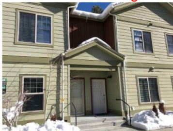
SJV E Building
