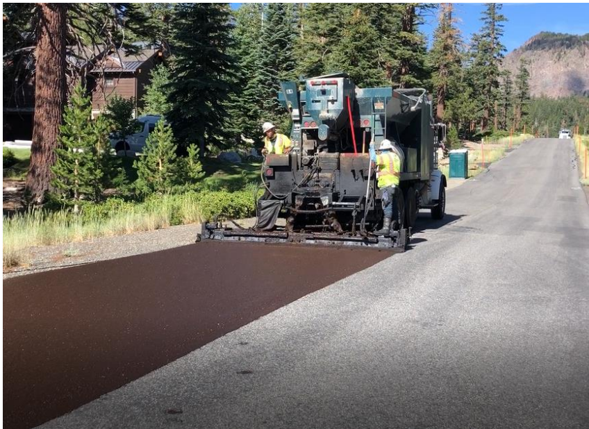
Application of the slurry seal
