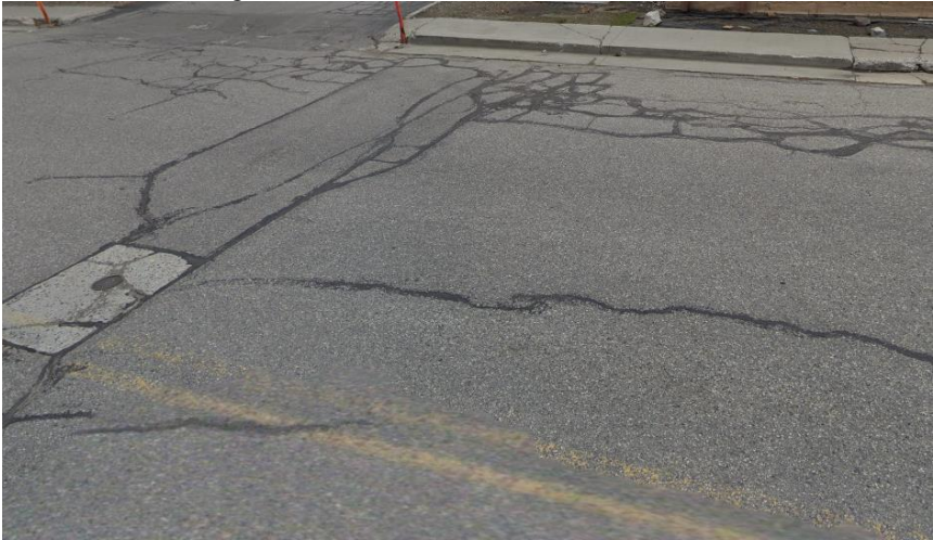
Severe road cracking and curb deterioration
