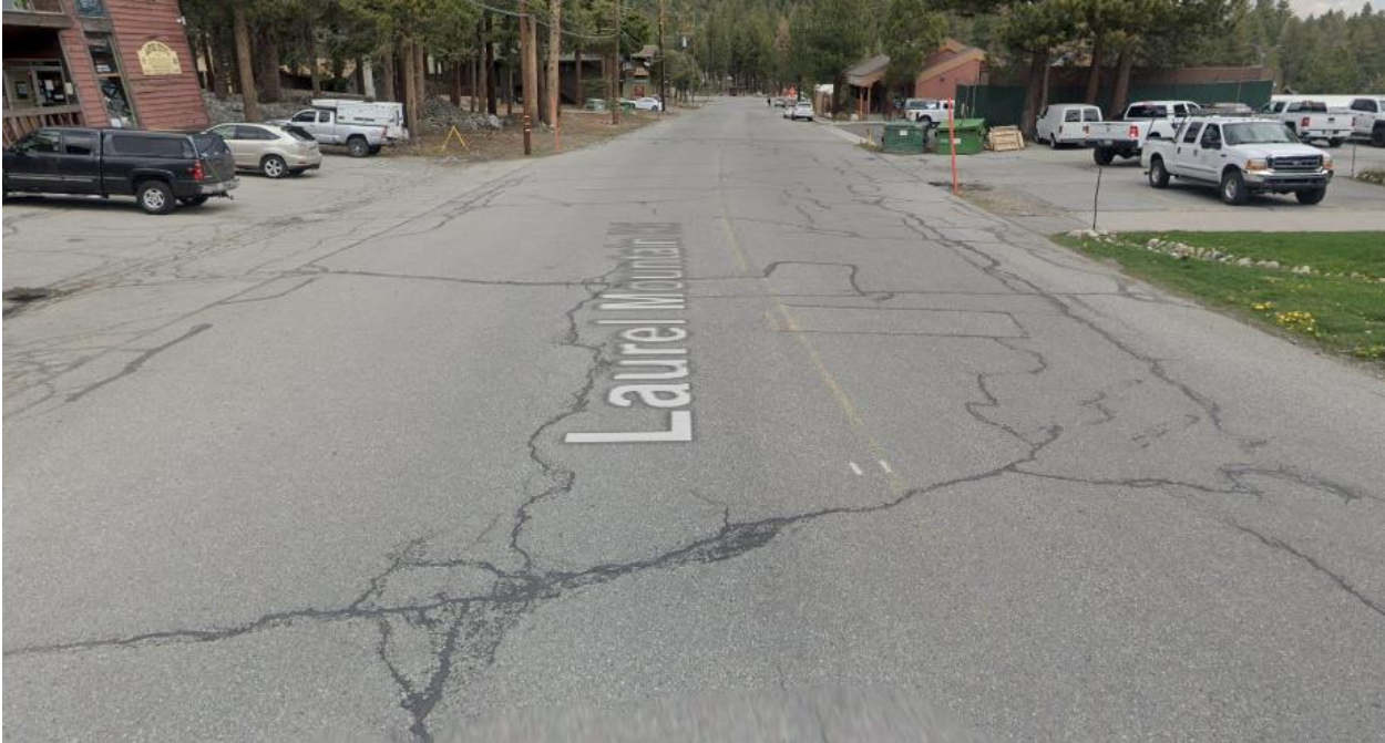
Severe road cracking and curb deterioration
