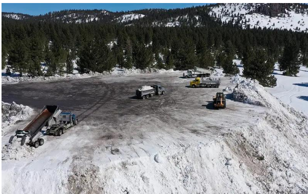
Figure 5: Snow trucking operations unloading snow at the snow storage site.
