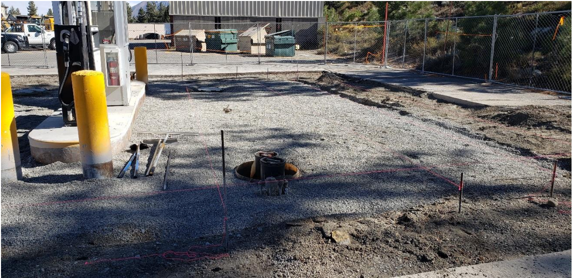
Grading gravel base in October 2023
