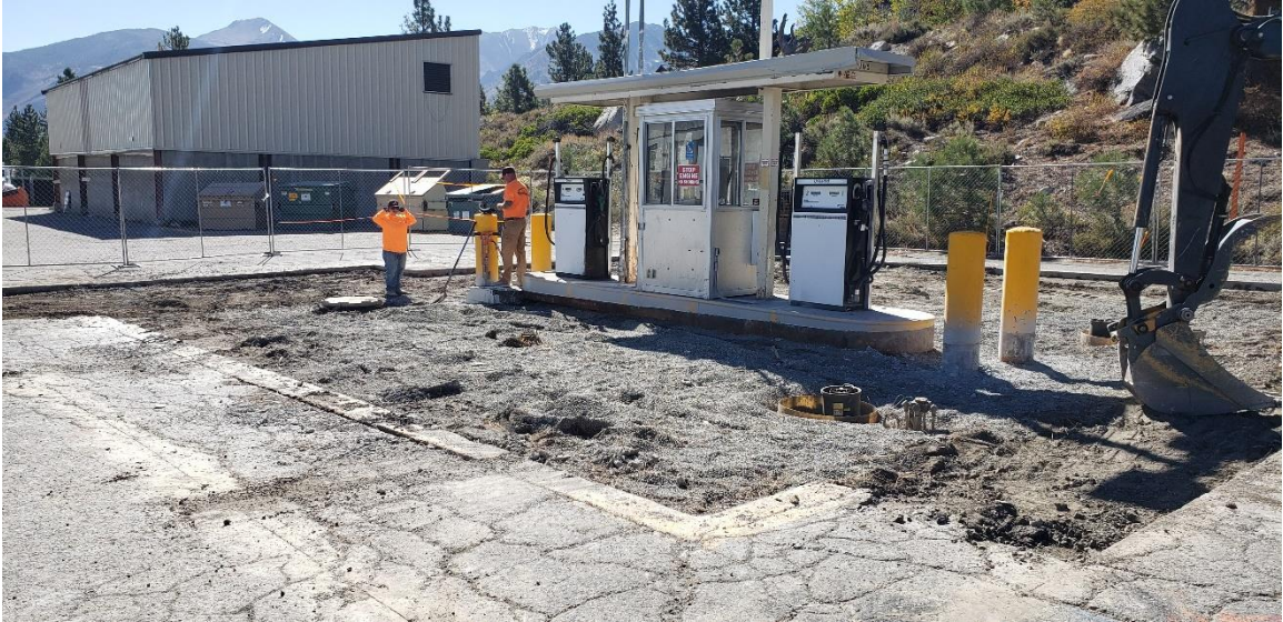
Demolition work in October 2023
