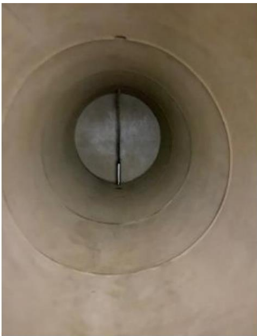
Before Lining, After Sandblasting
