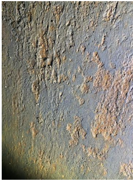
Internal wall before sandblasting
