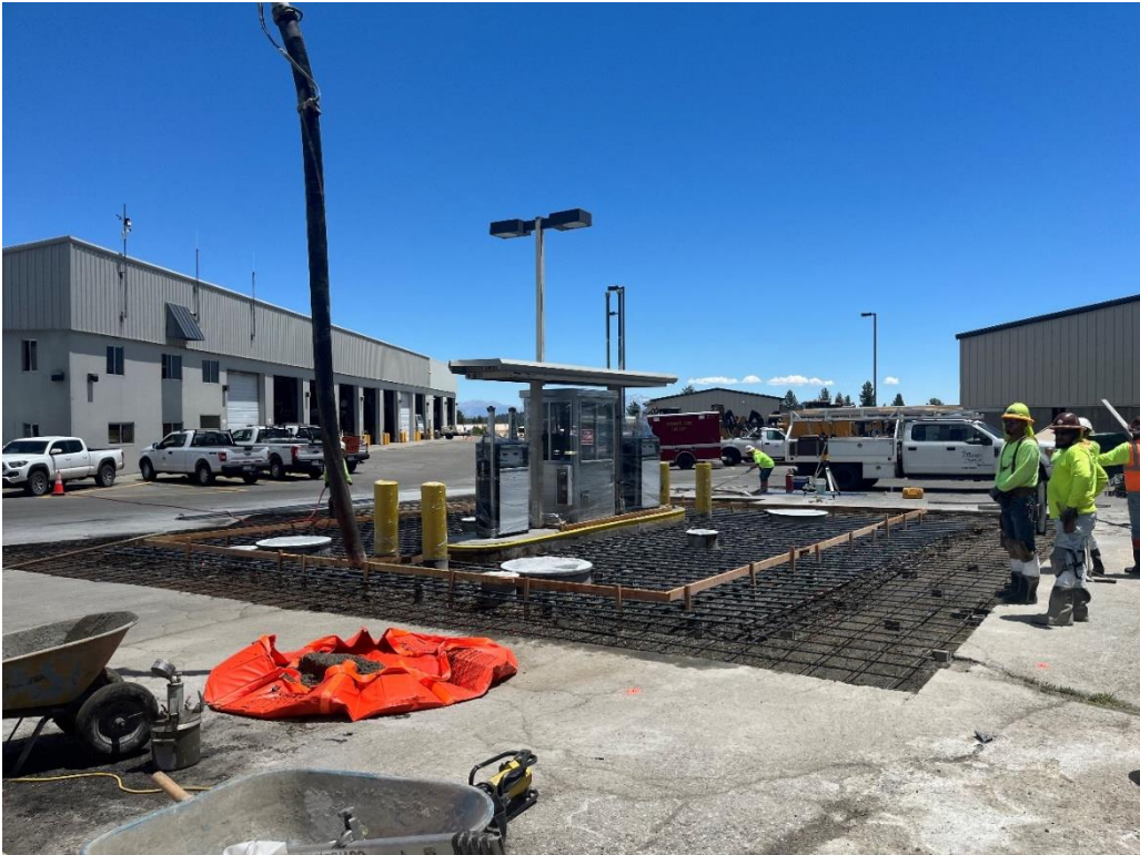
Pouring concrete in 2024
