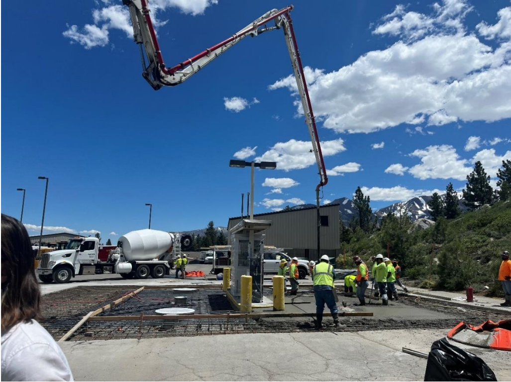
Placing concrete in 2024
