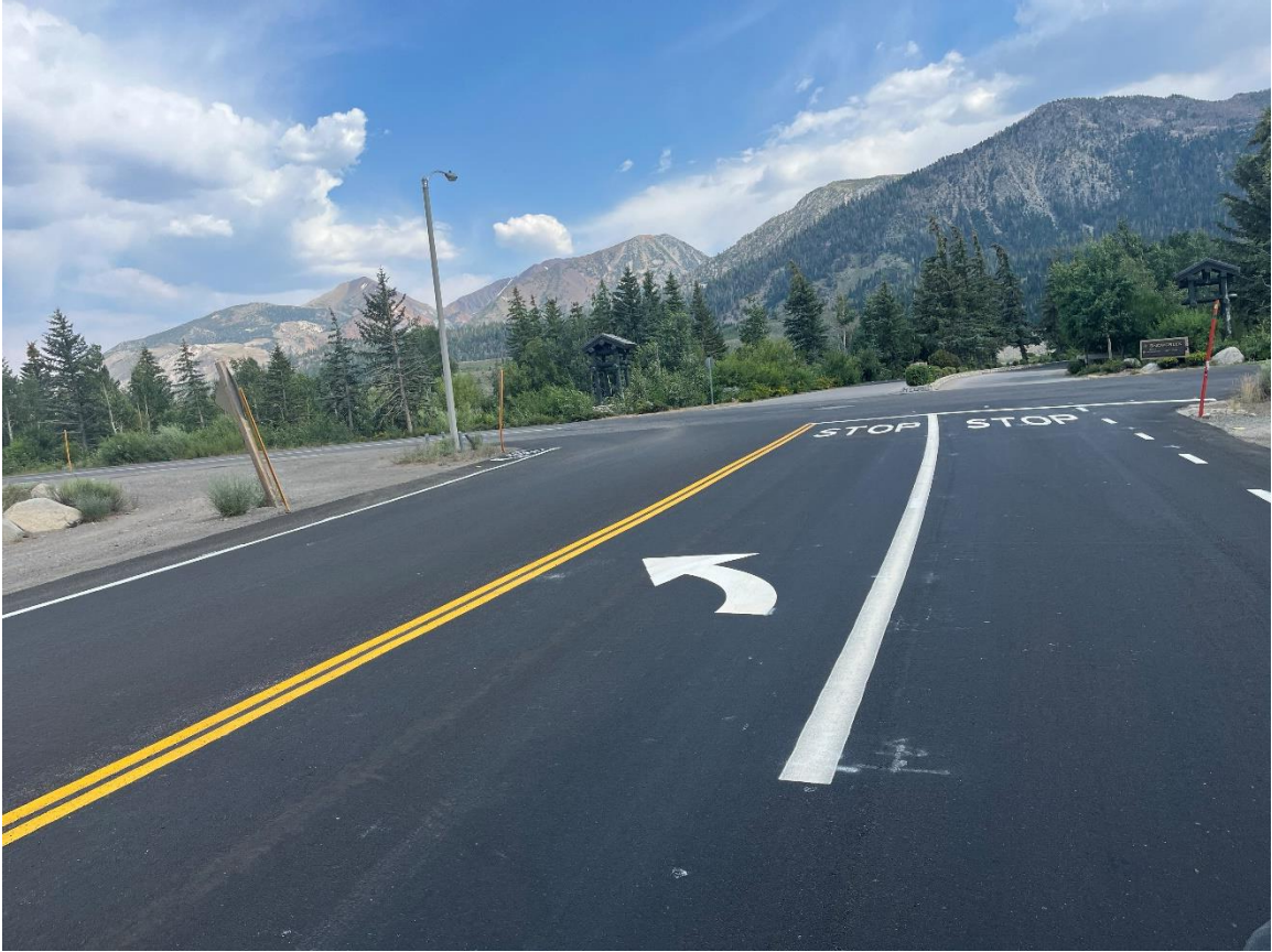
Striping and pavement markings after the slurry seal
