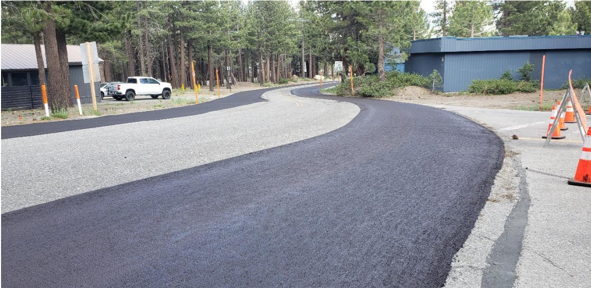
Application of the slurry seal along Forest Trail
