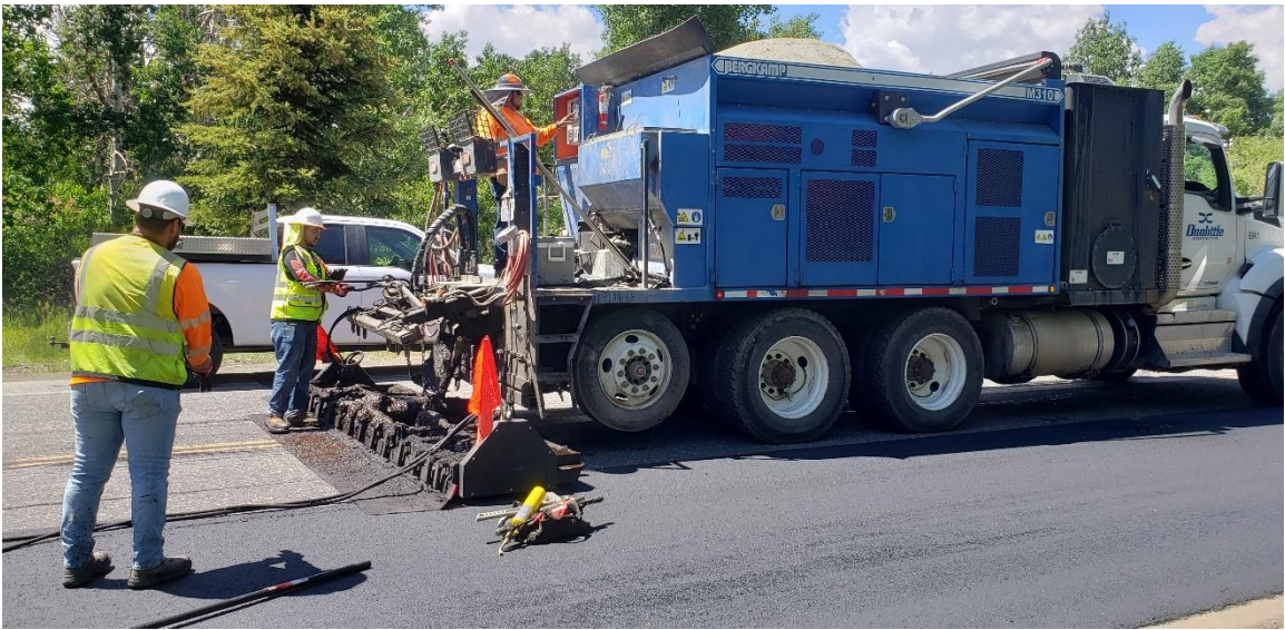
The specialized box truck required for a slurry seal. The machine mixes sand, aggregate and oil before laying material at a precisely measured thickness
